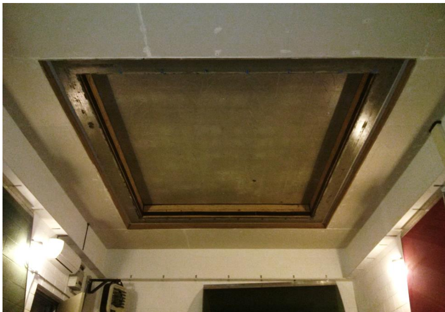
Receive Room View of Test Specimen Installation
