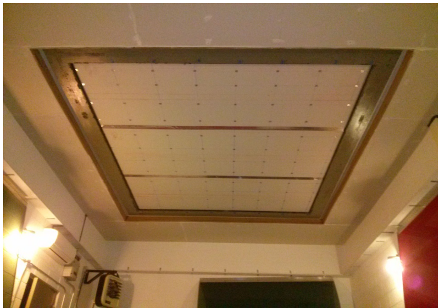
Receive Room View of Test Specimen Installation
