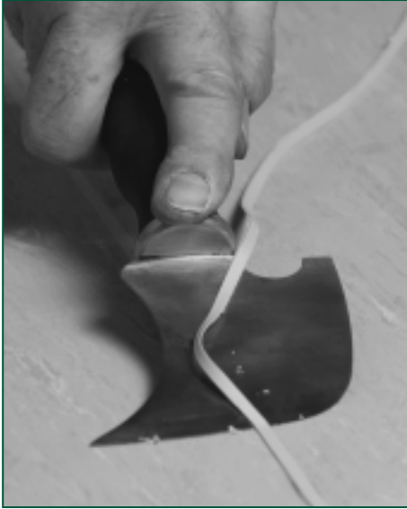
Figure 30 Final trim after the weld has cooled
