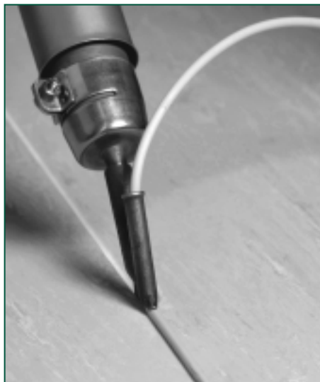
Figure 27 Applying the weld
