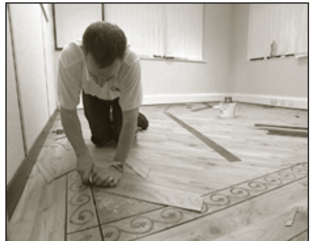
Installing border and perimeter tiles
