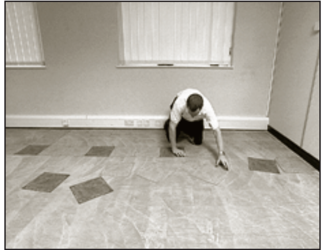
Loose lay tiles to check set out.
