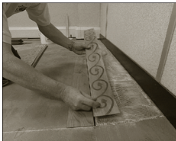
Setting out for border installation
