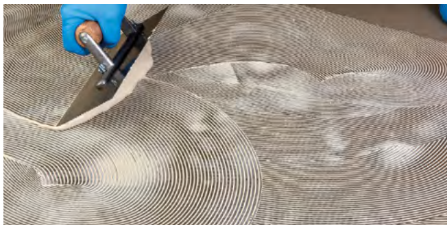
Figure 3.6 Spread the adhesive
