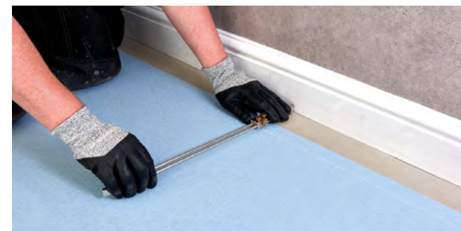
Figure 3.2 Scribing the wall profile
